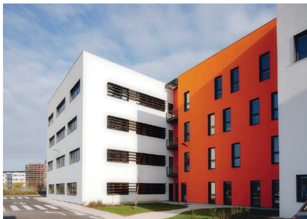
The new premises in Valence are BBC certified.
